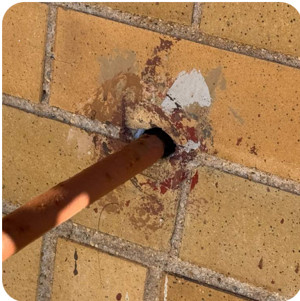
Cement spalling and internal rust
