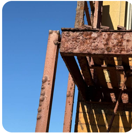
Leg support disconnected due to severe rust jacking - Imminent Safety Hazard
