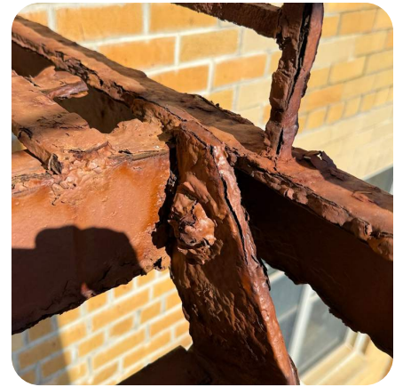
Corroded Stringer connection
