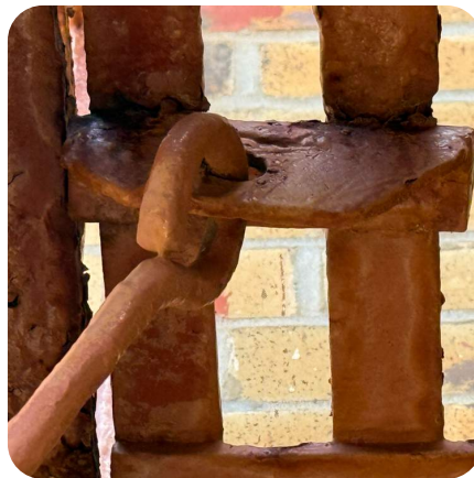
Ladder's release mechanism suspect with internal rust
