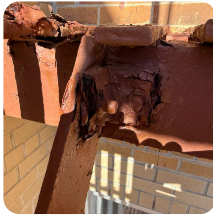
Corroded Stringer connection
