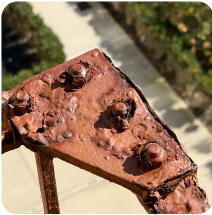
Corroded rail gusset plate connection
