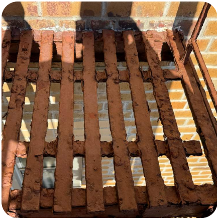
Corroded Platform slats
