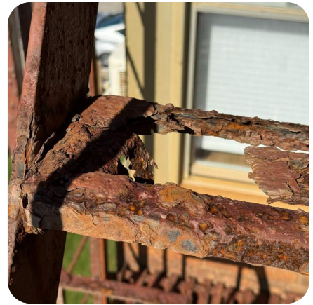
Severely corroded Tread - Life Safety Concern
