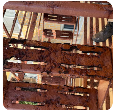
Corroded Tread - Imminent Danger
