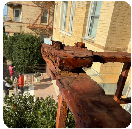
Corroded rail gusset plate connection with rust jacking
