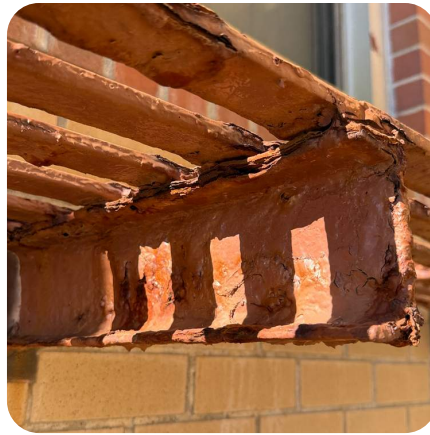
Corroded slat connections
