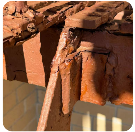
Corroded Stringer connection
