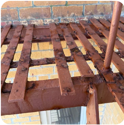
Missing & Corroded Slats - Imminent Danger
