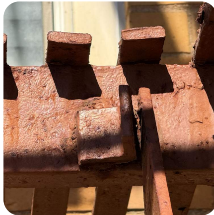
Corroded Stringer connection
