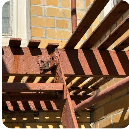
Corroded Stringer connection
