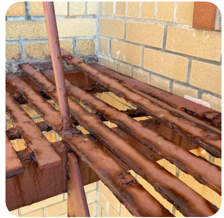
Corroded slat connections, detached - trip hazard
