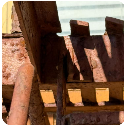
Corroded Platform slats
