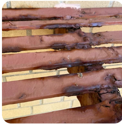
Corroded slat connections
