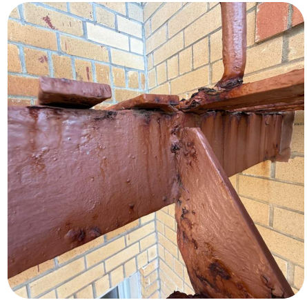
Suspect welded stringer connection. Missing bolted clip connection.
