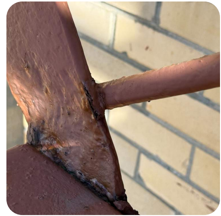
Corroded stringer, railing & tread connections
