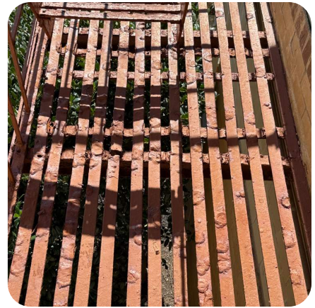
Corroded slat connections, detached - trip hazard
