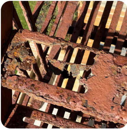
Severely corroded Treads - Life Safety Concerns & Imminent Safety Hazards
